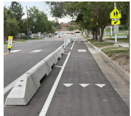
CHURCH AVENUE PROTECT BIKE LANE USING THE SAFE-T LANE DIVIDER.
