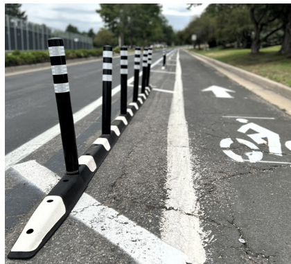
BELLEVUE AVENUE PROTECT BIKE LANE USING THE ORCA LANE SEPARATOR.
