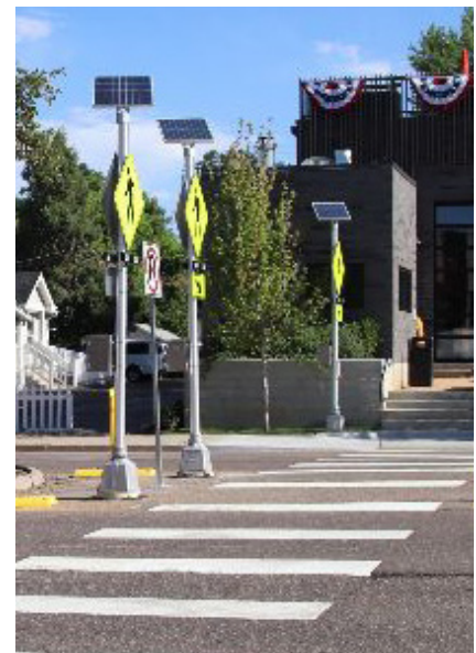
RAPID-RECTANGULAR FLASHING BEACON (RRFB) PEDESTRIAN CROSSING INSTALLED ON LITTLETON BLVD.
