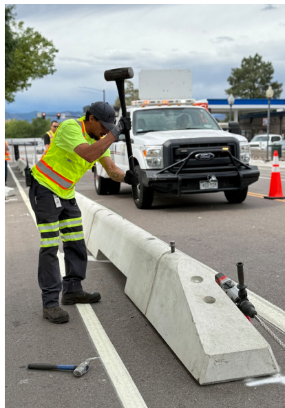
LITTLETON OPERATIONS CREW INSTALLING THE SAFE-T LANE DIVIDER ON CHURCH AVE.
