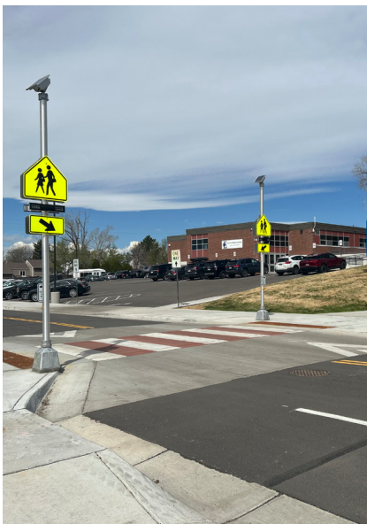
RAISED CROSSING AS PART OF PHASE 1 OF THE EUCLID AVENUE RECONSTRUCTION.
