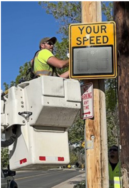
OPERATIONS CREW INSTALLS SPEED FEEDBACK SIGNS NEAR A SCHOOL.
