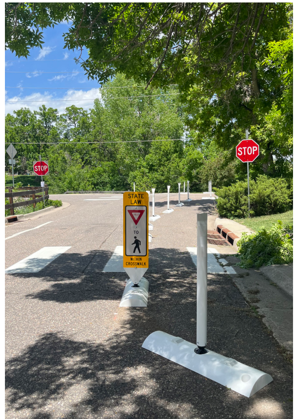
CURB EXTENSION PILOT PROJECT AT LAKE AVENUE AND STERNE PARKWAY INSTALLED IN 2024.
