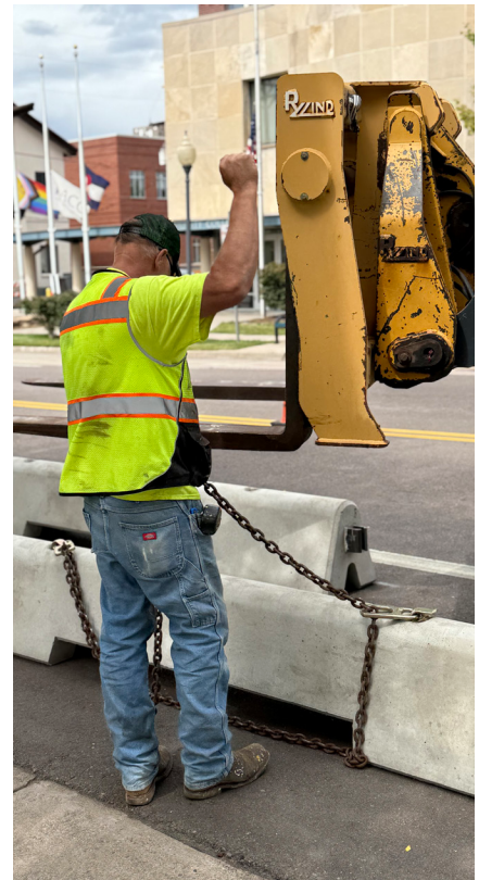
OPERATIONS STAFF INSTALLING THE SAFE-T LANE DIVIDERS ALONG CHURCH STREET.
