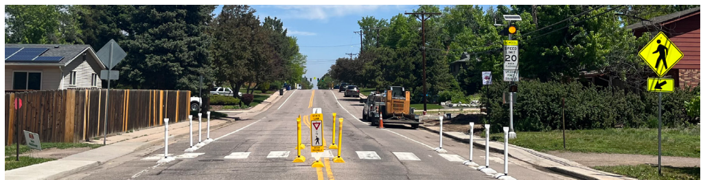
TEMPORARY CURB EXTENSIONS AND PEDESTRIAN MEDIAN ISLAND AT LEE GULCH TRAIL AND ELATI STREET.
