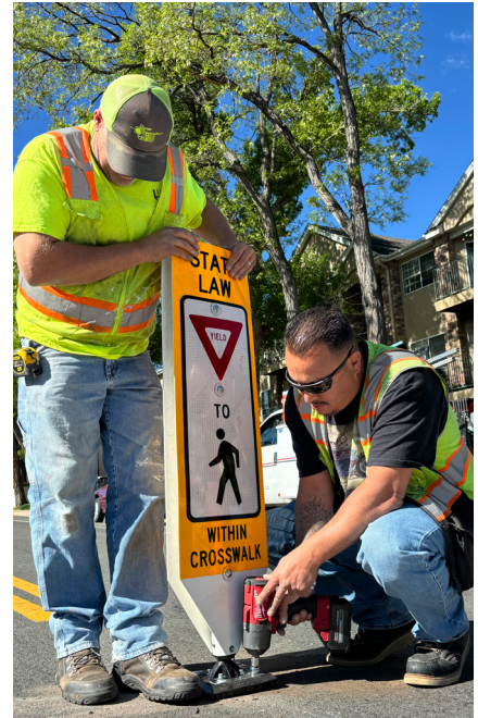
OPERATIONS STAFF INSTALLING IN-STREET PEDESTRIAN SIGNAGE.
