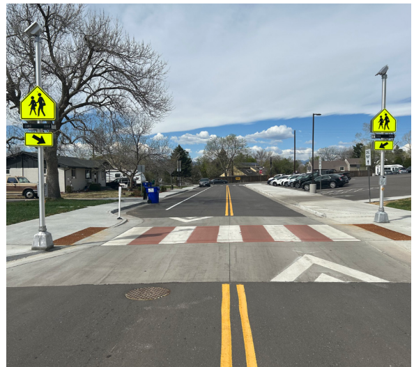
RAISED PEDESTRIAN CROSSING INSTALLED AS PART OF THE EUCLID AVENUE RECONSTRUCTION PROJECT PHASE 1.
