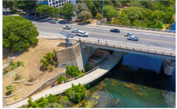
Figure 13. Trail underpass in Austin, TX
