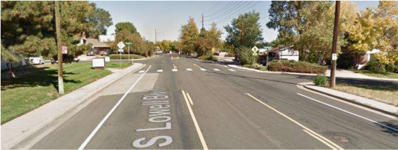
Lowell Blvd and Aksarben Ave (south of Arrowhead Rd)
