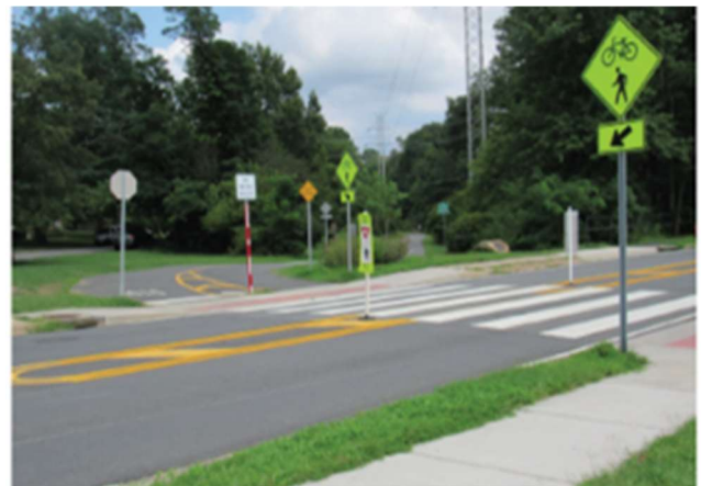
Figure 2. Markings and warning signs at a W&OD Trail crossing in Vienna, VA
