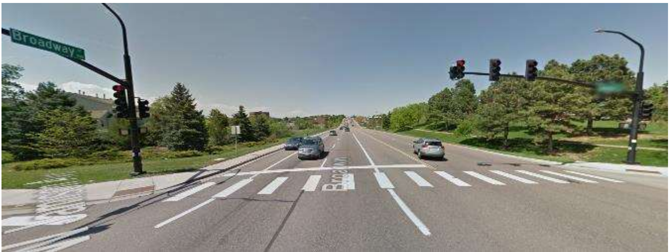
Broadway north of Jamison Ave (tunnel)
