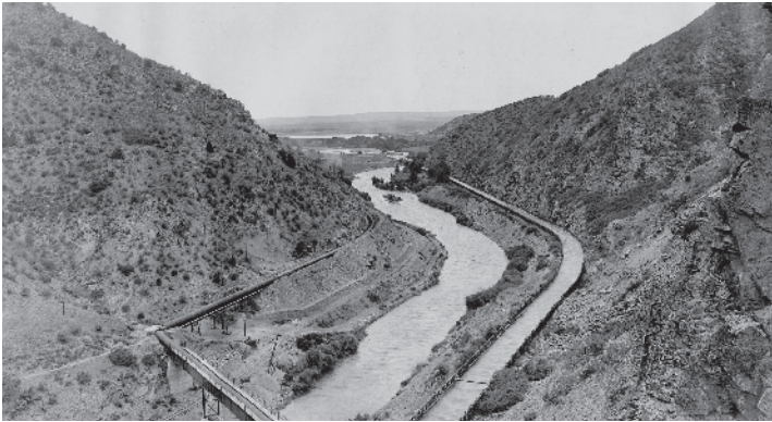
The Start of the Canal in Waterton Canyon
