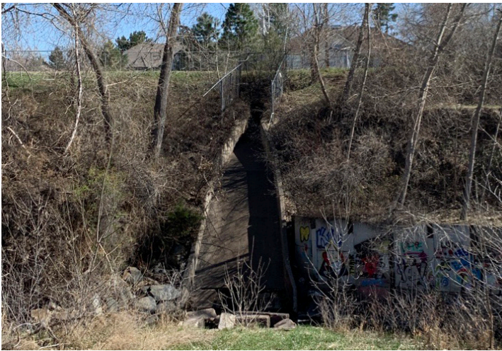
Little Dry Creek Waste Gate
