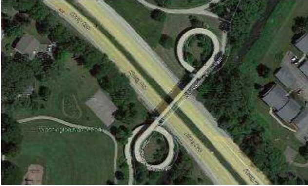
Figure 12. Trail overpass in Madison, WI
