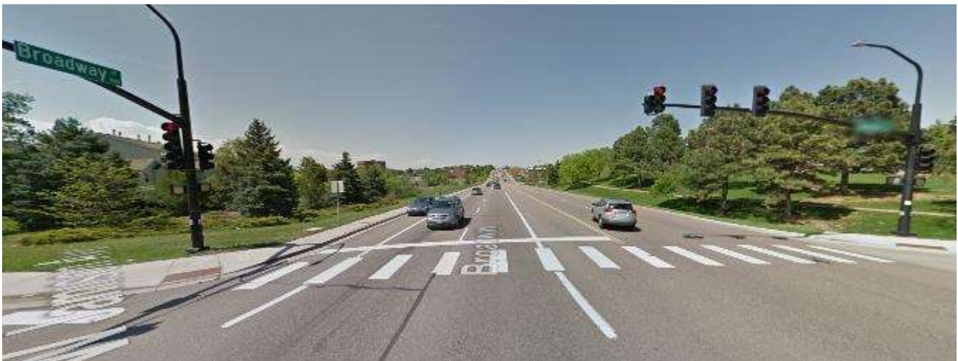
Broadway north of Jamison Ave (tunnel)
