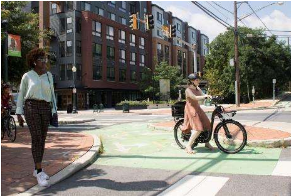
Figure 11. Protected Intersection in Silver Spring, MD
