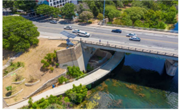
Figure 13. Trail underpass in Austin, TX
