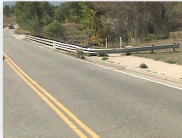
Discontinuous Sidewalk along County Line Road near the Highline Canal Trail
