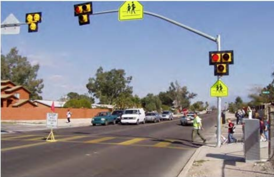
View of a HAWK Signal Installation
