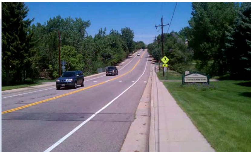
Lee Gulch Trail crossing at Prince St, looking north. Notice the sag vertical curve.
