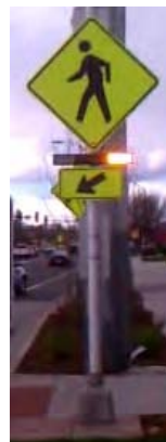
Activated Pedestrian Crossing with RRFB, Boulder, CO
