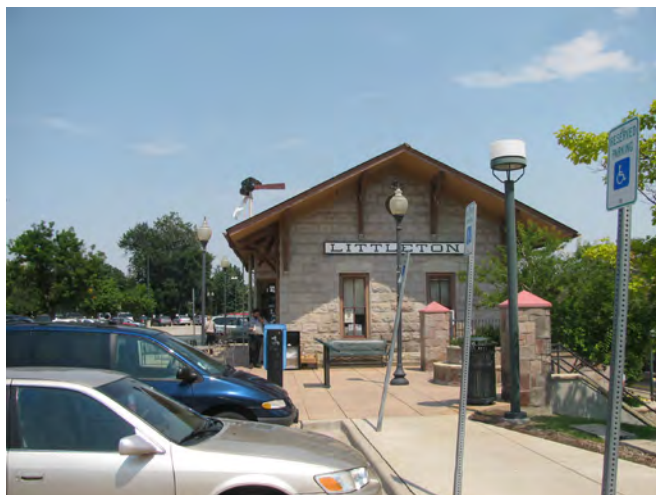
Image 12. Littleton RTD Light Rail Station
