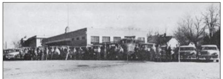
This view shows the south and west elevations of the 1952 warehouse building as it appeared in 1955 with the then-current fleet of equipment. Photo: Courtesy of IREA, from the 1955 Annual Report .
