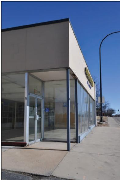
The well-designed International Style Goodyear Auto Service Center is an example of a master design commissioned by Goodyear from an unknown architect. The T-shaped building has a planar sense for enclosure, with extremely thin walls as compared to building's bulk. The brick end-walls bracket a glass curtain wall on the boulevard side, and set back behind the driveway, a row of aluminum and glass garage doors.
