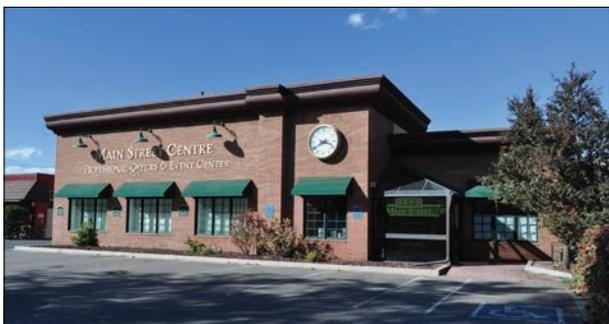
The former CeBuzz Super Market was originally a plain-walled functional structure with a projecting wing wall that rose above the roofline, now partially demolished. To better blend with the older buildings downtown, it was re-clad and an over-sized cornice and traditional-style clock were added. In the 1970s, the former supermarket was occupied by the *Littleton Independent*, founded in 1888, the sole justification for the significance of the building.
