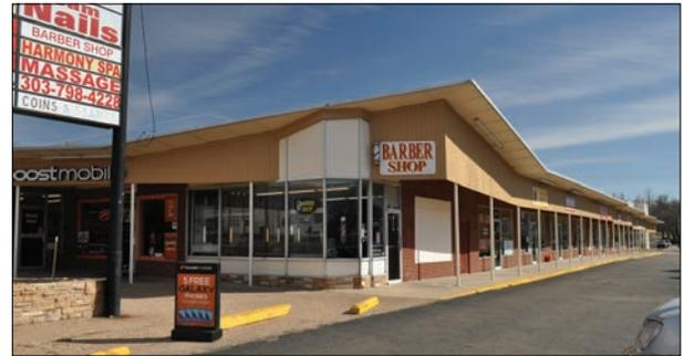
This Modernist red-brick and glass curtain-wall strip-mall has a distinctive cantilevered roof line that rises in a wedge at the northwest corner. The arcade of shops, sheltered by an integral canopy supported by steel pilotis, runs south perpendicular to the street. The handling of the relationship of the brick to the fenestration, and the prominent use of those unadorned piloti in the Woodlawn Shops, resembles the lost original appearance of Woodlawn Shopping Center.
