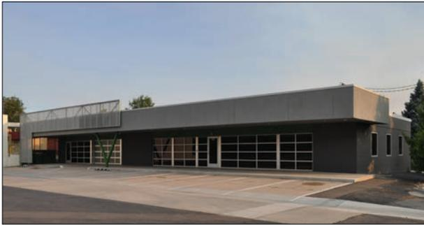
Originally Moore's Restaurant, this was probably a builder's design. It is nominally Modernist with its simple rectilinear form, flat roof, and boxed cantilevered-eave sheltering the front. Though the building retains these defining elements, in 2017, it was completely resurfaced and the fenestration and entry were reconfigured. Currently the building appears to be contemporary with all its period elements covered or removed.
