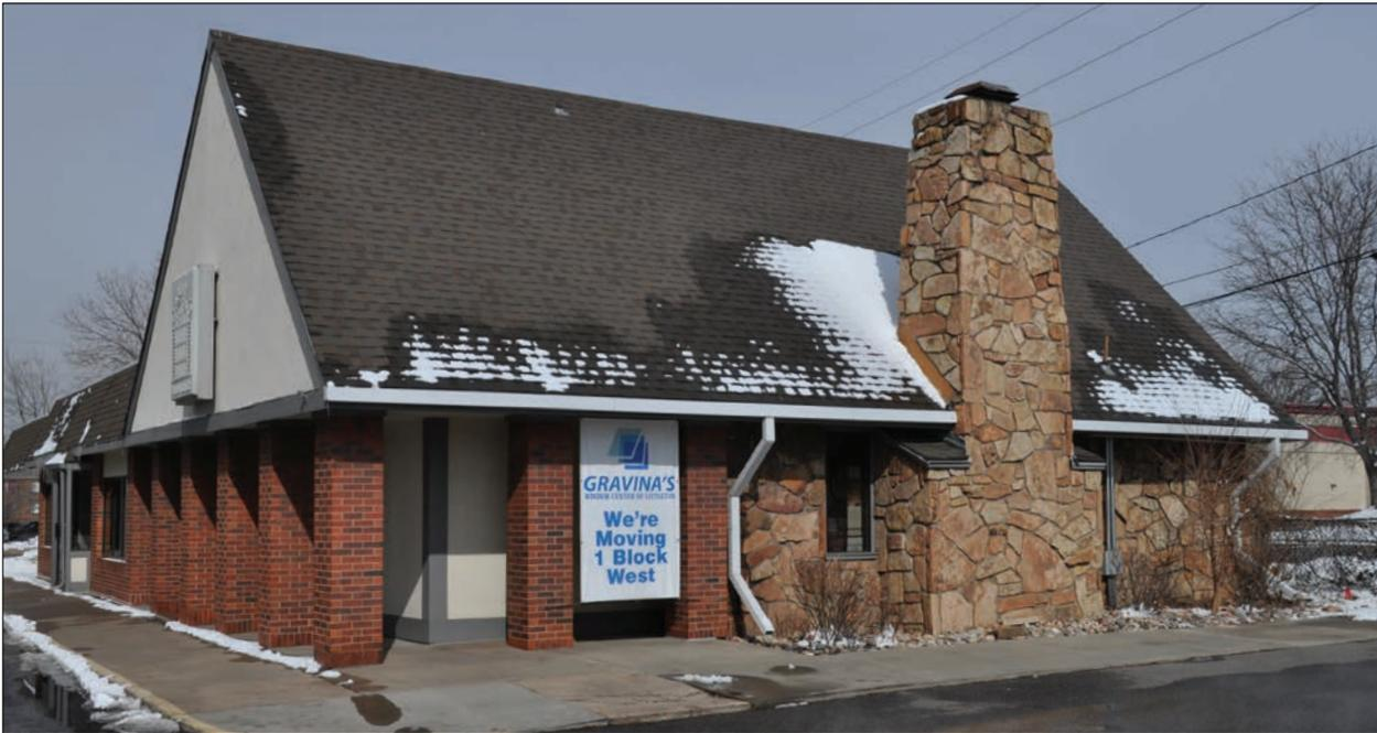
The Rustic Modernist Style Brock's Eating House is defined by its enormous gabled roof sitting heavily on thick brick pillars. This oversized gable has been based on an equilateral triangle, and is connected to a long low brick wing that has a mansard style canopy. A noteworthy feature on the boulevard side is the monumental chimney in expertly-laid field stone, the familiar form scaled up to match the gigantic roof shape.
