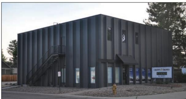
A kit for a warehouse building of no particular distinction that was assembled from prefabricated parts. A much more ambitious and thoughtful version of a building that was similarly constructed with manufactured elements is the Dawson & Company Realty Office Building at 609 West Littleton Boulevard, in Tier Two of this survey.
