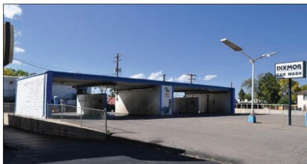
An extremely simple structure comprised of a roof and side walls divided into two bays with four car-washing stalls and open at both ends. Cars drive through the bays with drivers wash their vehicles using coin-operated machines. Despite its stripped-down character, it is an elegantly conceived design. The car wash retains its "space-age" free-standing lamp standard. Car washes, like gas stations, illustrate the importance of the automobile in the postwar era.
