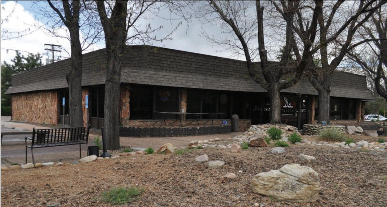
A handsome low-profile building, the Hasty House Restaurant, by an unknown architect, embodies the characteristics of Rustic Modern Style architecture. It has a broken gable eyebrow roof canopy that functions as a mansard. The walls of the building are made of expertly laid field stone, locally known as “moss rock”, that frame horizontally-oriented picture windows in smoked glass on the front facade, and continuing onto the side walls.
