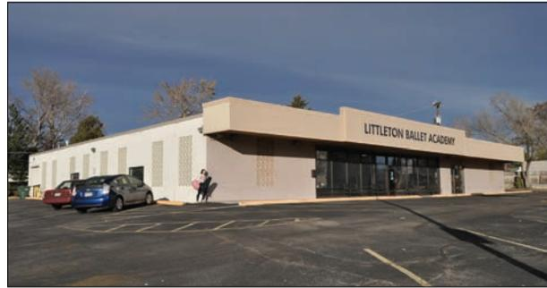
A simple box with a flat roof, the Shoppers Mart was originally a single large retail store. Modernist in style, the building's simplicity is somewhat relieved by the glass curtain wall entrance, and by the generous use of concrete block grills over large vertical windows. The boxed-in overhanging canopy that runs across the front has been somewhat altered, to its detriment.
