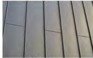
STANDING SEAM PRIMARY (SECONDARY IN ULUC)
