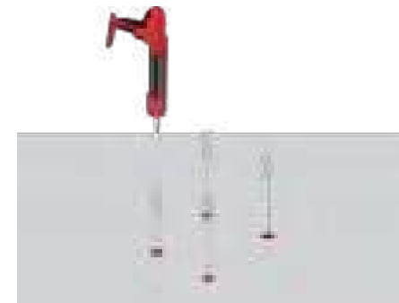
Figure 4 - Inject the resin.
