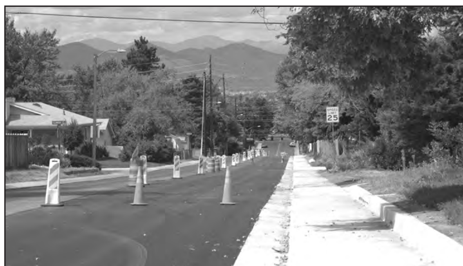
What will one million dollars buy? The rehabilitation of Powers Avenue from Windermere east to Broadway. The project included a wider sidewalk on the north side, traffic calming circles on the 16-block stretch, and a smooth new surface.
